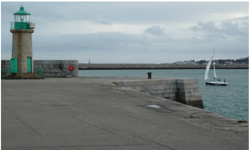
Figure 5.8.7: The West pier harbour entrance light looking towards the East pier
