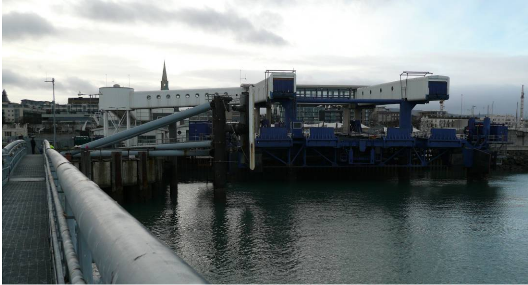
Figure 5.8.4: The HSS ferry berth looking back towards the town
